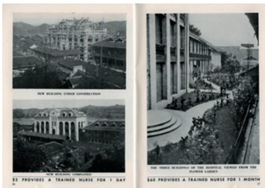
Fig. 1. Yuanling Catholic Hospital (from Your Yuanling Catholic Hospital).
